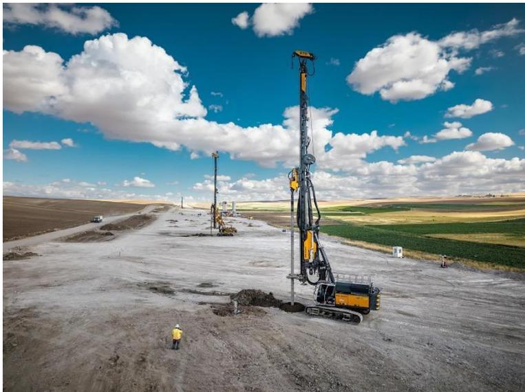
(1) Resource-efficient single column mixing method: The existing in-situ ground is mixed with a binding agent, single columns are produced after hardening.
